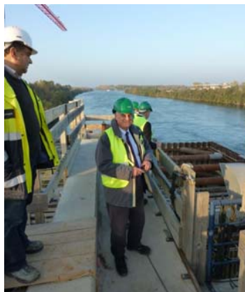
Giles Chichester at the Iffezheim Hydropower plant.
