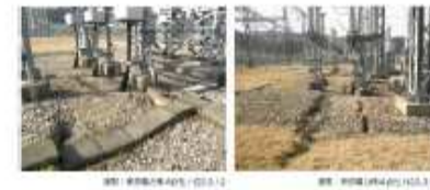
Yoronomori line, Cable in substation (subsidence)
