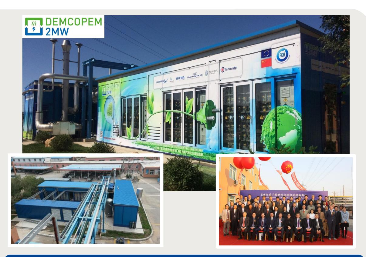
2MW plant at Ynnovate, Yingkou (province Liaoning), China Design, build and operate a 2 MW power generator, with full integration of heat and power with an existing chlorine production plant. Fully automated way of operation and remote control DURATION: 2015-2018 with FCH JU Funding: ~5.5M€
